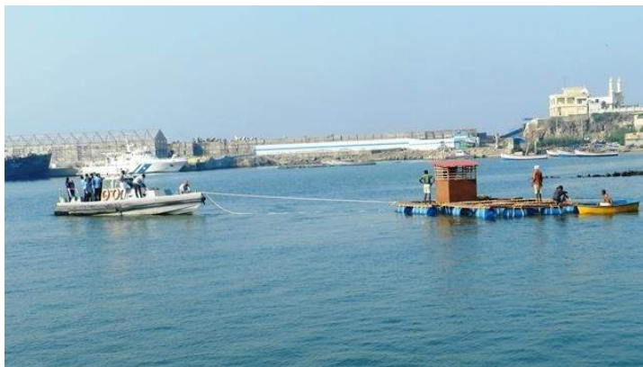
Towing the cage unit to mooring site
