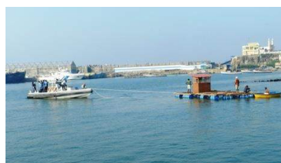
Towing the cage unit to mooring site
